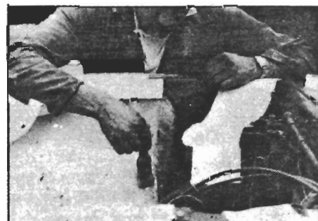
Laminating inside the engine bay joint. 1oz (300gm) mat is being used.
